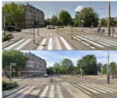
Removal of traffic lights on Alexanderplein
